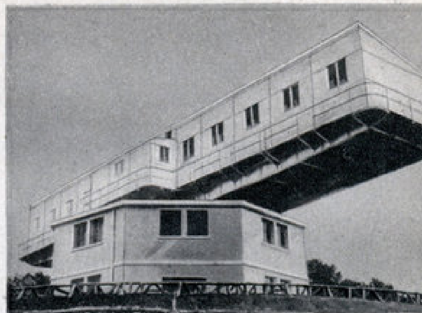
The most up-to-date hospital in France is this weird-looking structure near Cannes. The upper half revolves to face the sun all day long to give patients the benefit of the rays.
